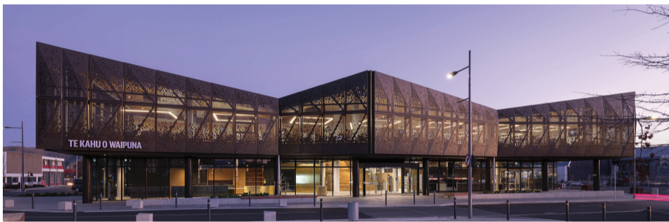
Te Kahu o Waipuna has won the public architecture category in the Te Kāhui Whaihanga New Zealand Institute of Architects Local Awards. Credit: Barry Tobin
