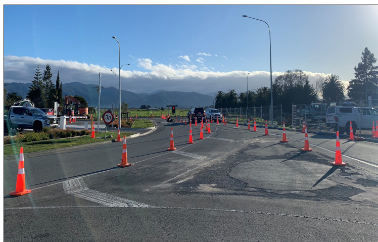
☑ Work has begun on a new roundabout at Marlborough Airport
