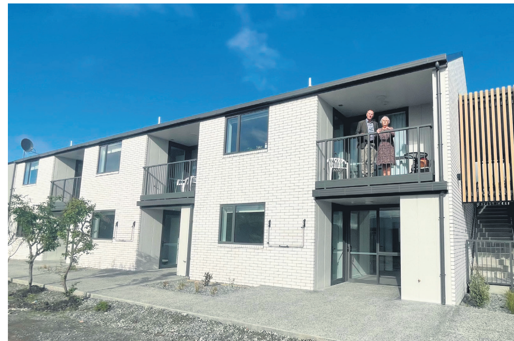
New 85 George Street tenant Sue Macdonald and Councillor David Croad enjoy the view from Council's first two storey units recently completed
