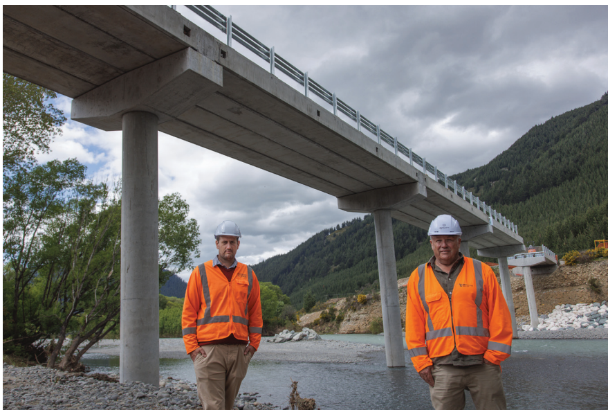
Councillor Scott Adams (left) and Steve Murrin at the bridge in the Waihopai Valley
