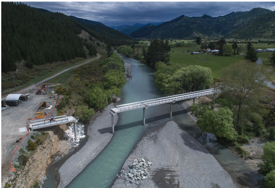
The nearly complete new bridge from the air
