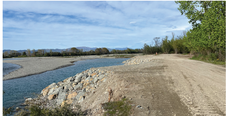
Completed groyne repairs on the Wairau River
