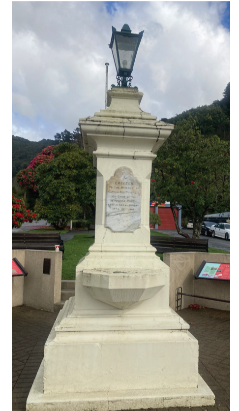
The Ronga Memorial in Havelock before recent repairs
