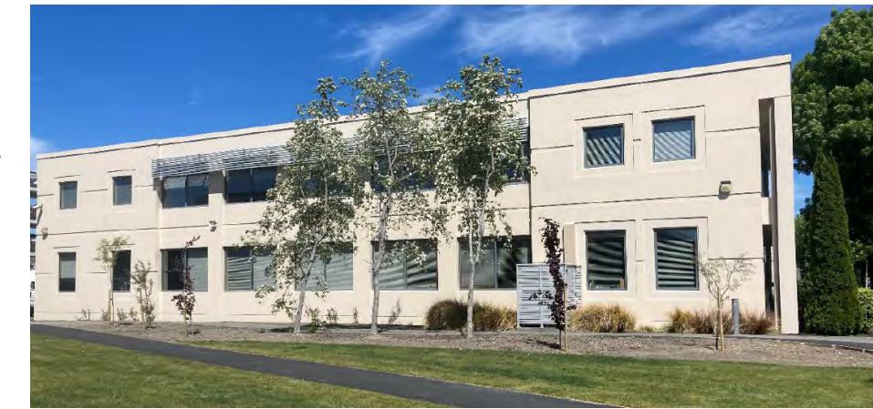
Three dogwoods are thriving following the demolition of the former Millenium Art Gallery and Council gardeners are now planting trees and shrubs in the area
