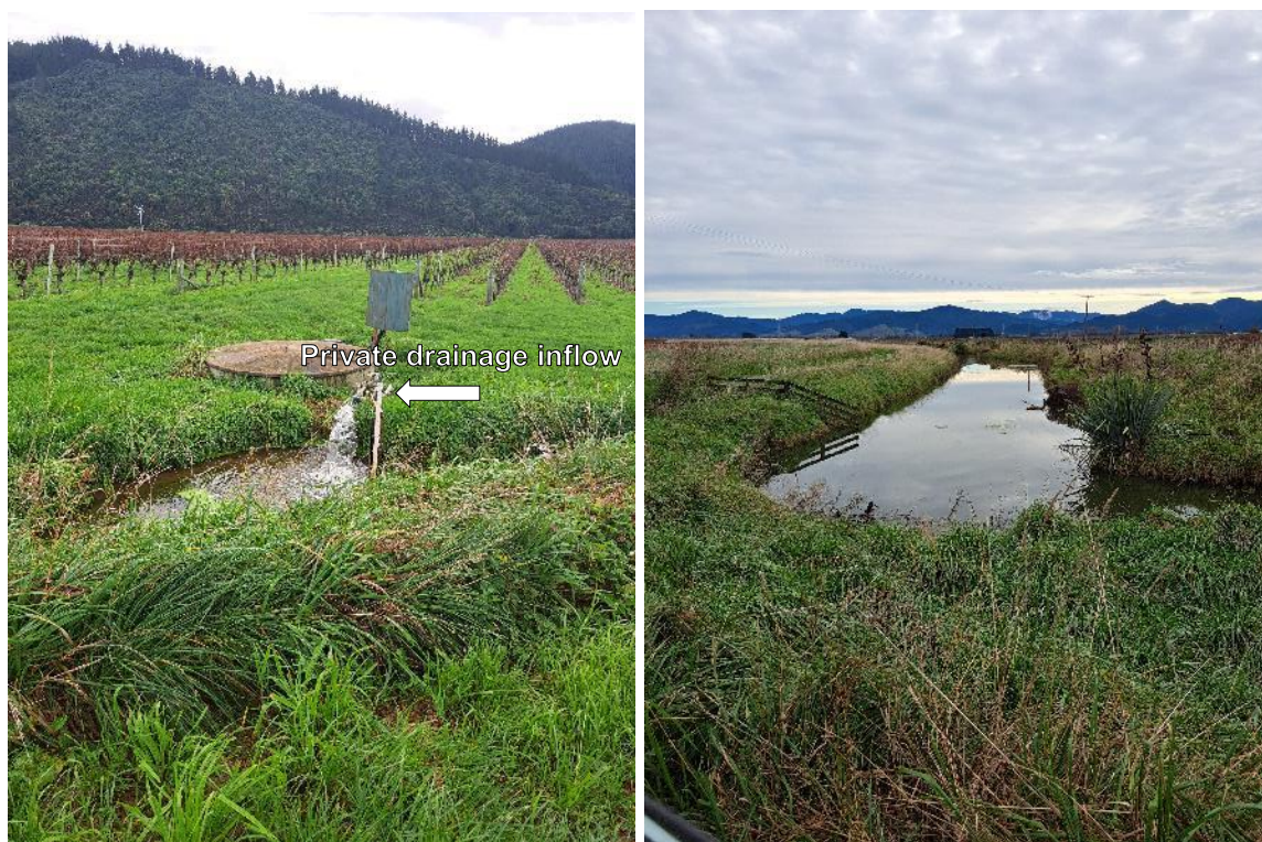
Figure 3-13 Pickerings Drain (left) and Pembers Road Drain (right) as viewed from Pembers Road on 27/06/2023 showing how close the water table is to ground level. The pipe discharge into Pickerings Drain (left) is a constant inflow from private land drainage
