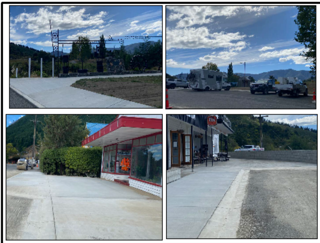
Figure 2 Canvastown Streetscape and Carpark - After
