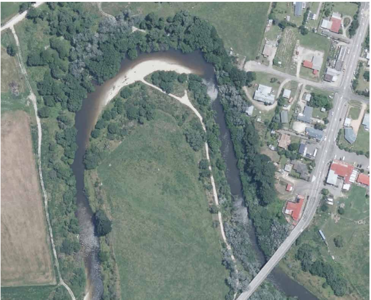
Figure E10 Pōrangahau River Channel Condition Prior to Event
