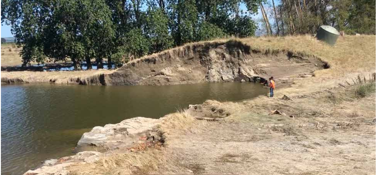
Figure 2.8 Ngaruroro Stopbank Breach Pakowhai 32
