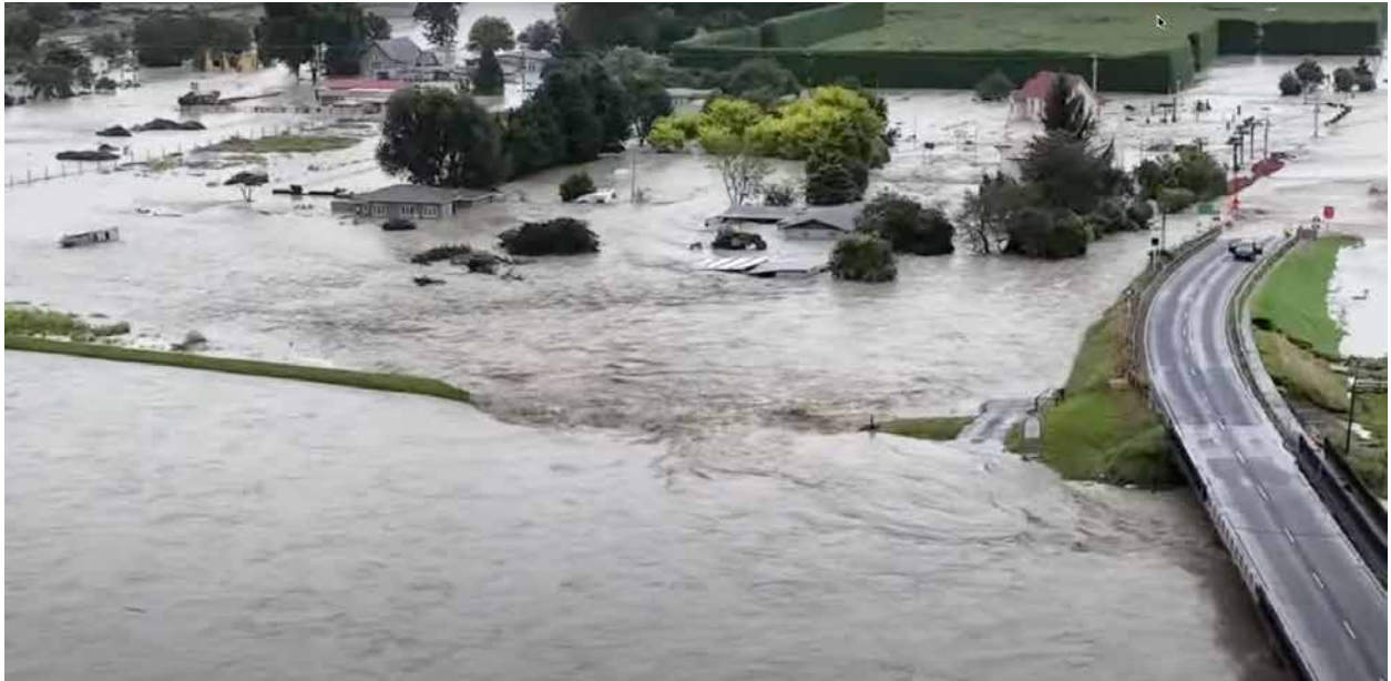
Figure 8.10 Ngaruroro River breach at Omahu 184
