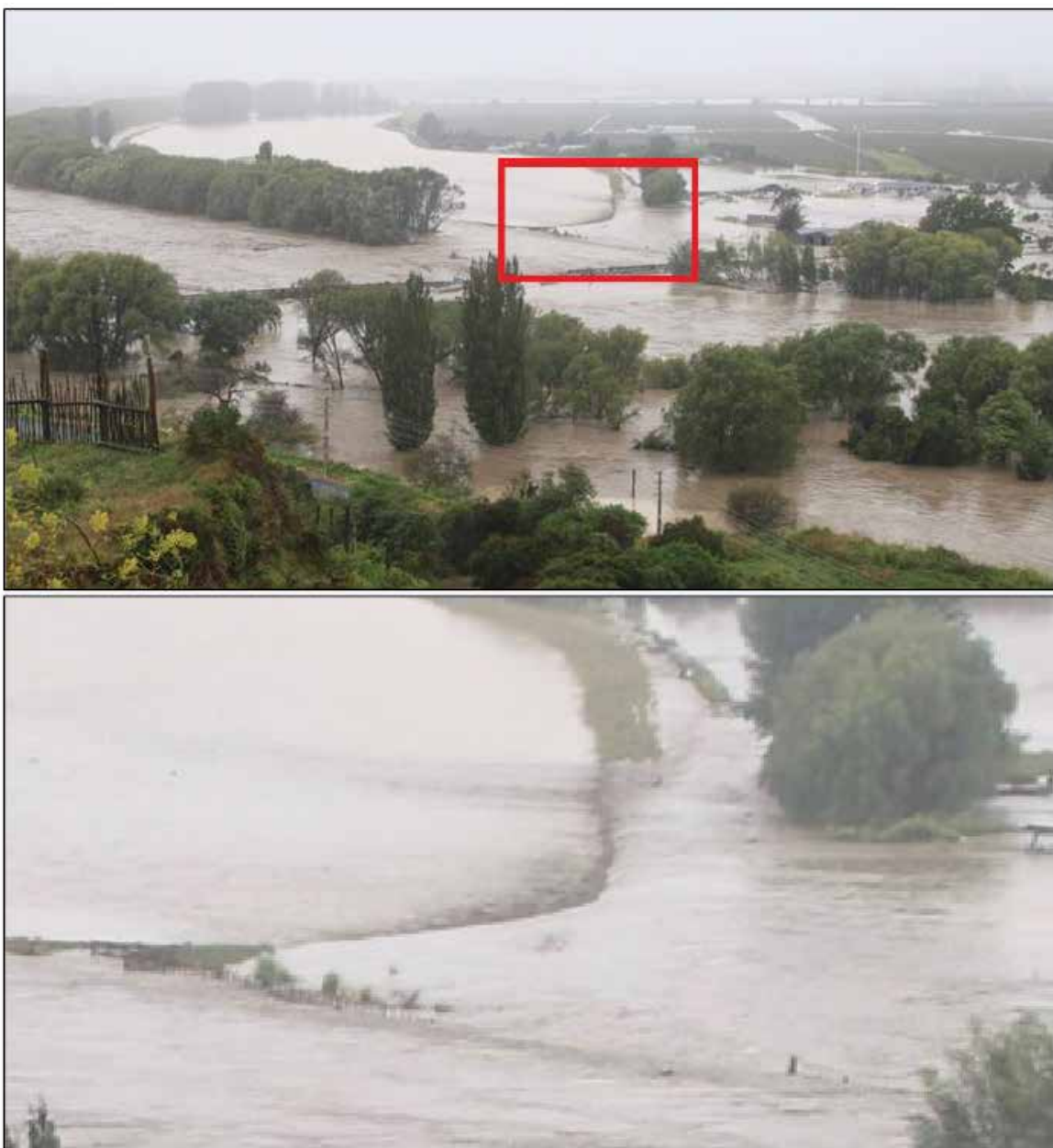
Figure 40.3 – Photos showing water flowing back into the Tutaekuri river at the approximate location of the designated breach site
