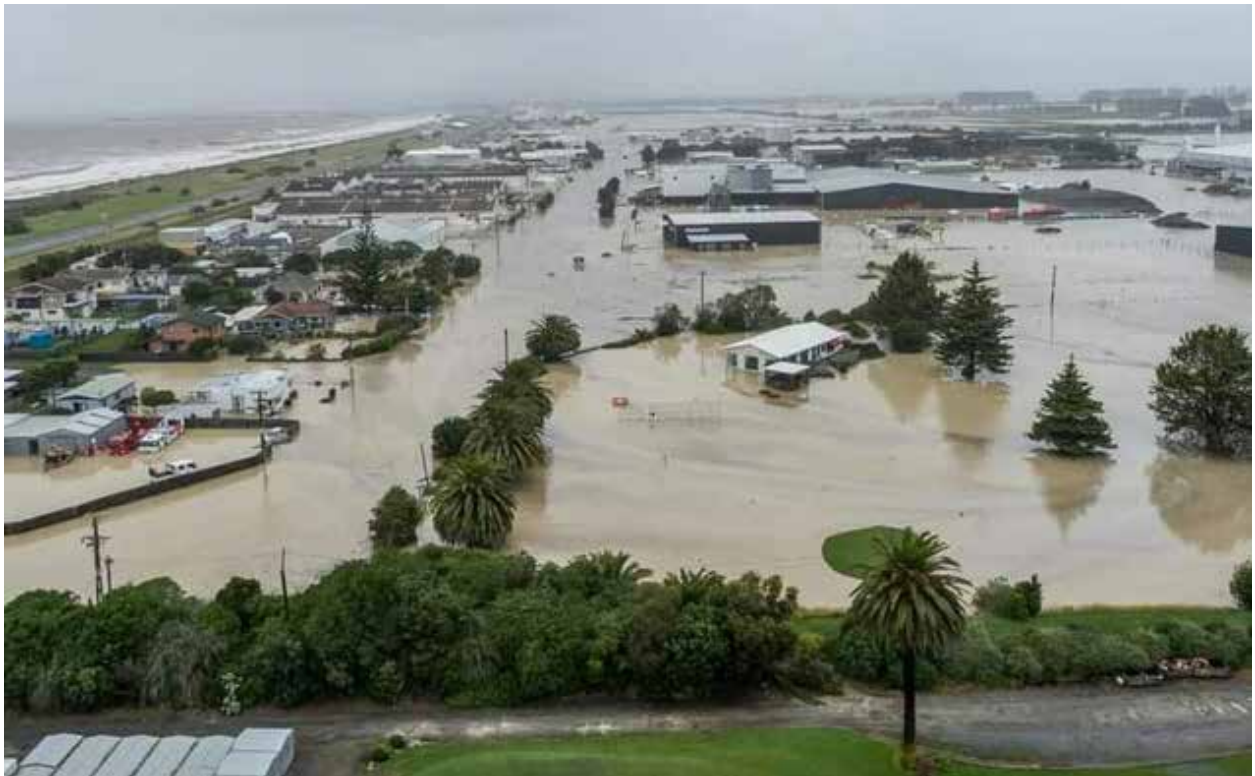
Figure 8.11 Breach at Awatoto 185
