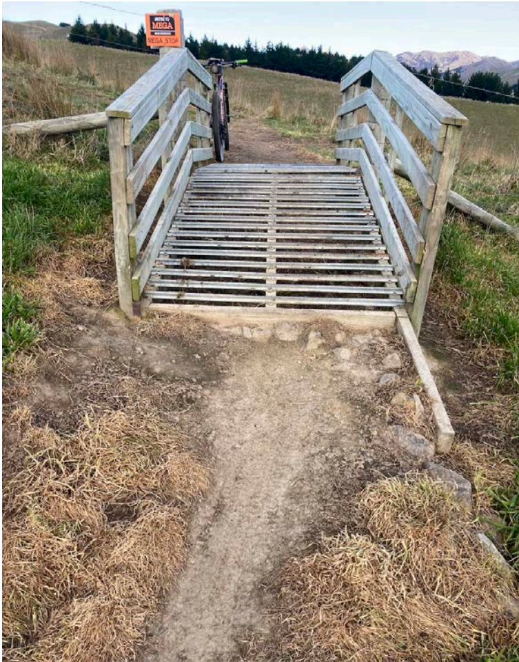
Figure 13. One of the trickier cattle stops heading uphill on Scenic Route (Northern)
