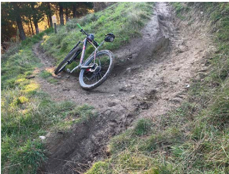
Figure 26. The badly eroded, tight and steep lower (second) corner on Mogwai. Some work could restore this to Grade 5 but probably not Grade 4, without realignment. Most importantly, the trail is eroding badly and is not sustainable.
