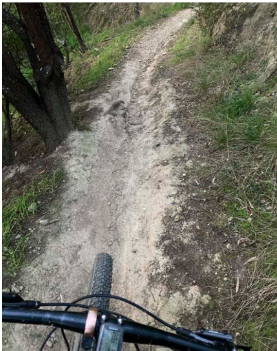
Figure 39. Part of Section 1 of Scenic Route (North). Not all of the formation is available to ride on. It's also rooty and stony with too-tight turns. Without realignment, the lowest grade this trail could be compliant with is Grade 4
