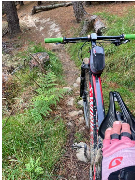
Figure 43. A stony section of Lamb Chops just below a very steep section. Much of the trail is unformed, as seen in the background, which is not sustainable for heavy use.
