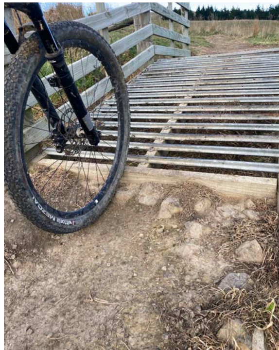
Figure 40. All of the cattle stops on Scenic Route are somewhat difficult to ride (and to walk). Lips, very steep ramps and tight approaches heighten the difficulty.
