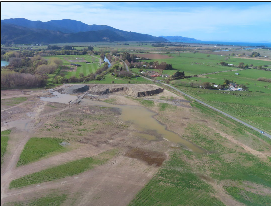
Figure 6 - Stockpiles, that will be hydroseeded
