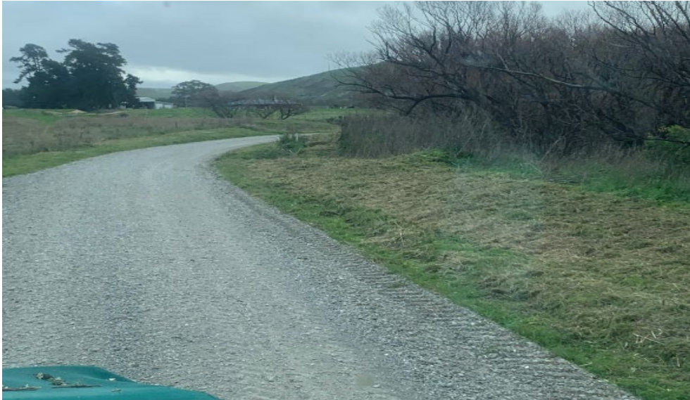
Figure 1 - Newly metalled and mowed Cable Station Road
