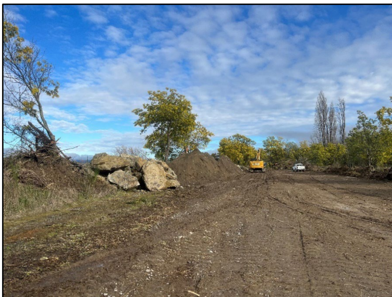
Figure 2 - Contractor Preparing Site
