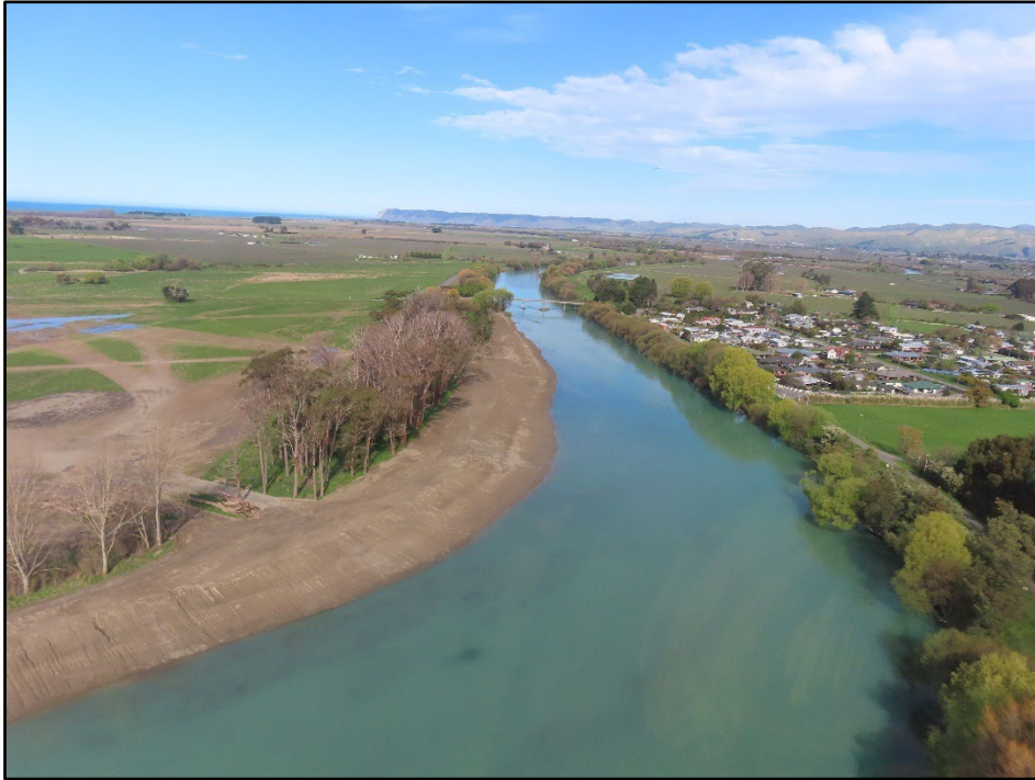
Figure 5 – Spring Creek Widening Project Stage 1 completed
