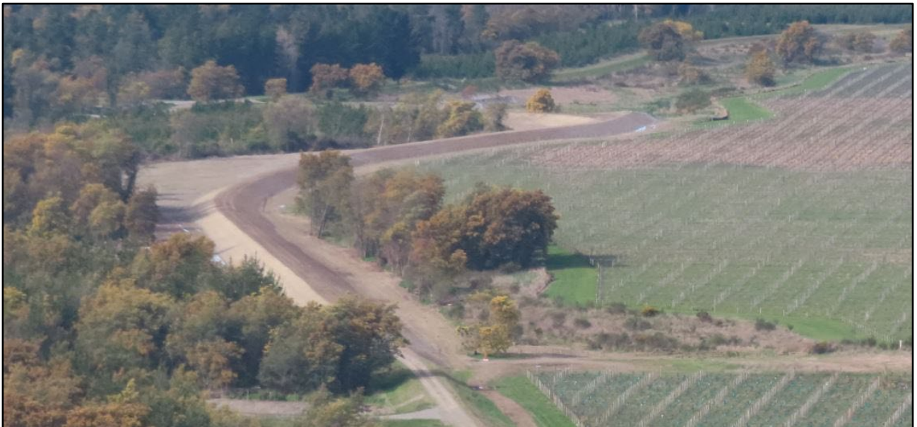
Figure 14 – new Condors stopbank realignment during the flyover
