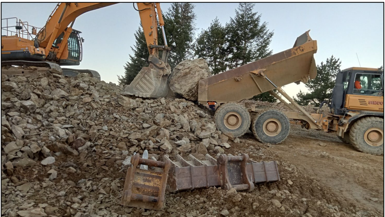
Figure 16 – toe rock from the top of the seam
