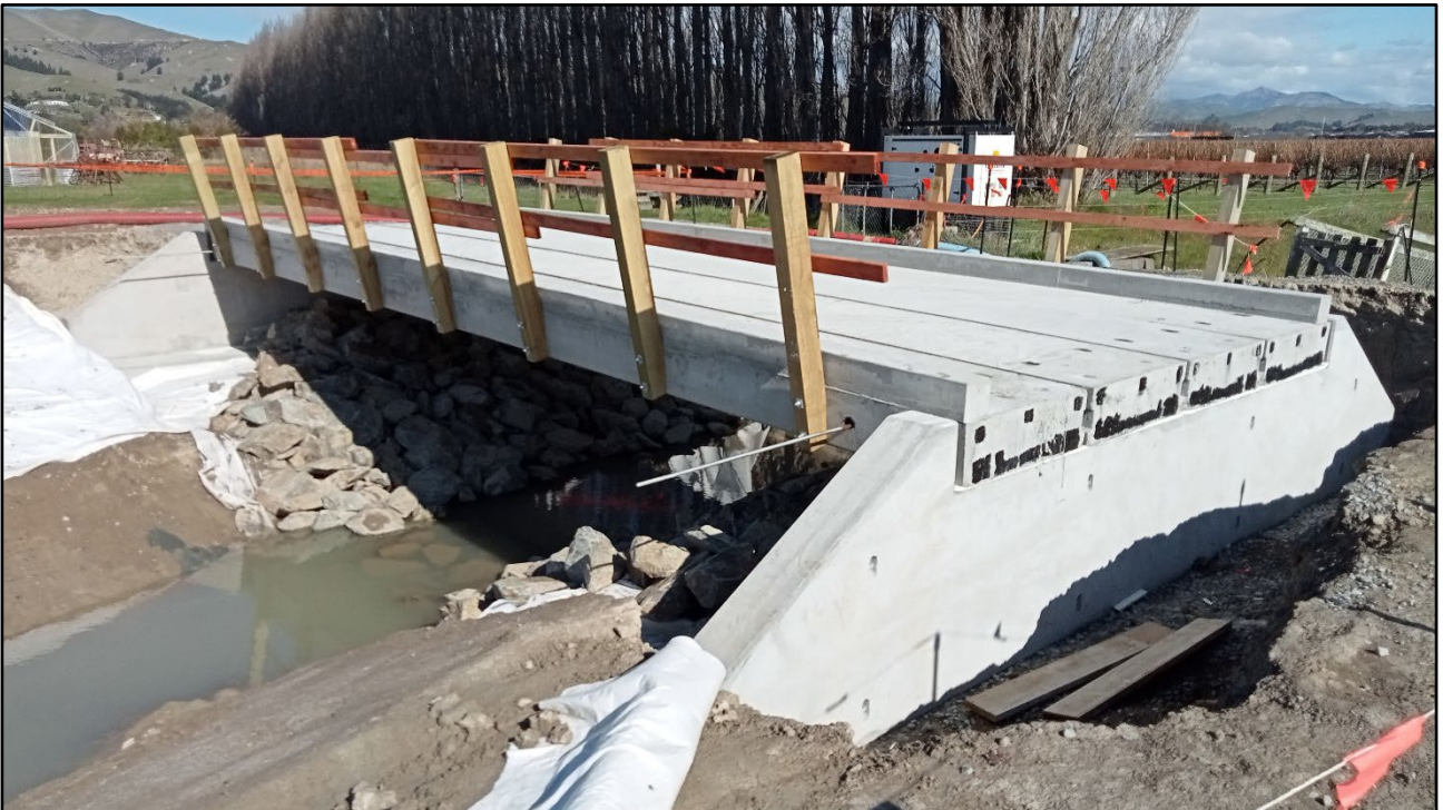
Figure 12 – Connor bridge construction
