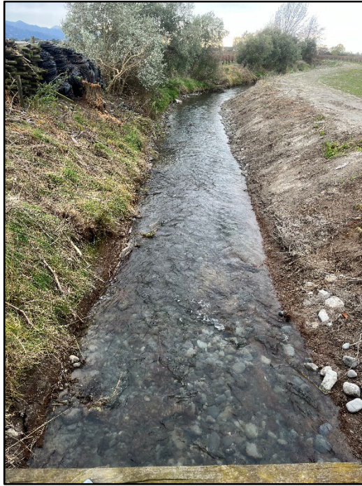
Figure 8 - Creek widening completed
