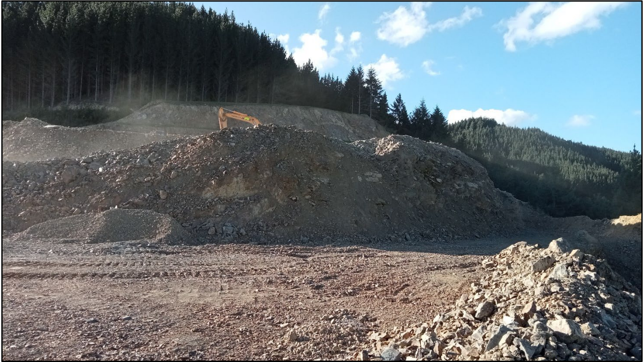
Figure 15 – Pukaka Quarry top bench working
