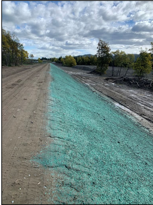
Figure 13 – new Condors stopbank hydroseeding
