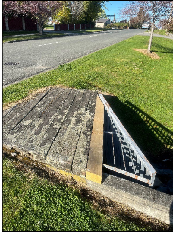
Figure 10 - Terrace Creek intake structure
