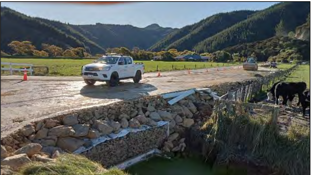
Figure 7 – extension and backfill of Quarry Drain Culvert complete.
