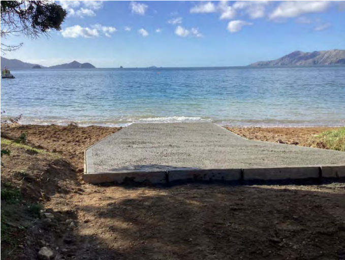
Figure 1 Concreting just completed on the French Pass Boat Ramp
