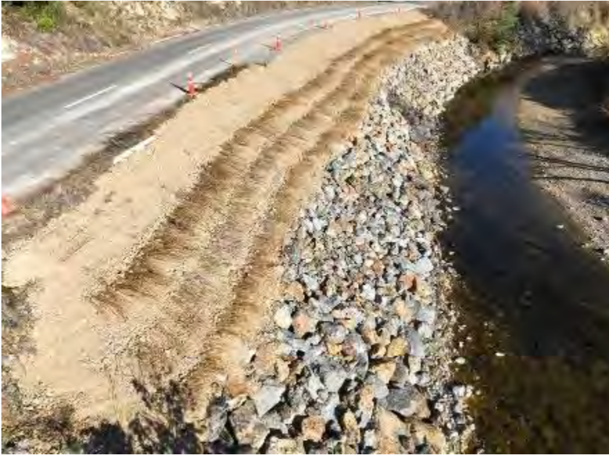
Brush wall completed at the Onamalutu Road scour site during – 30 May 2024.
