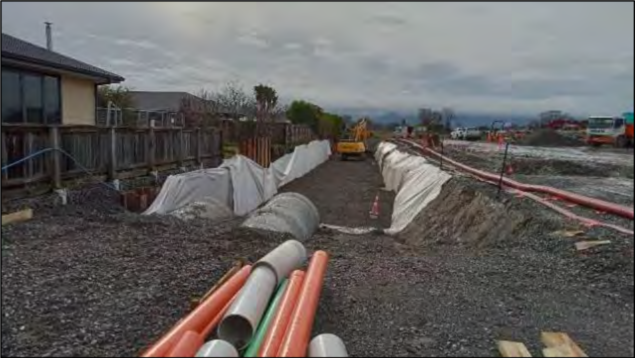
Figure 2 –Railway Drain Culvert bedding preparation for the final lengths of pipe.
