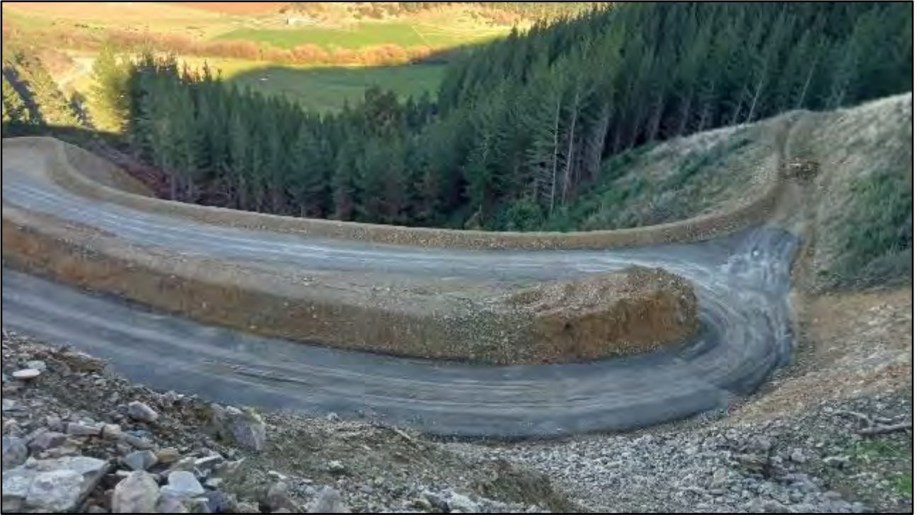
Figure 13 – Pukaka Quarry haul road switchback.
