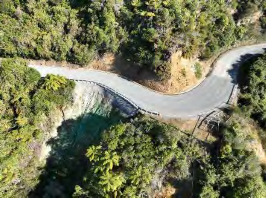
*Site completed on Queen Charlotte Drive at RP 07369 – 30 May 2024
