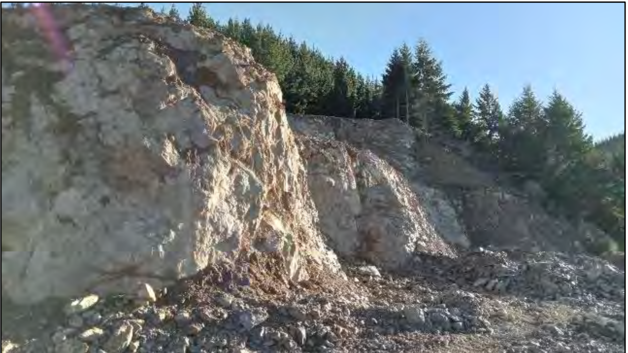
Figure 14 – Pukaka Quarry upper edge of rock seam being exposed for production.
