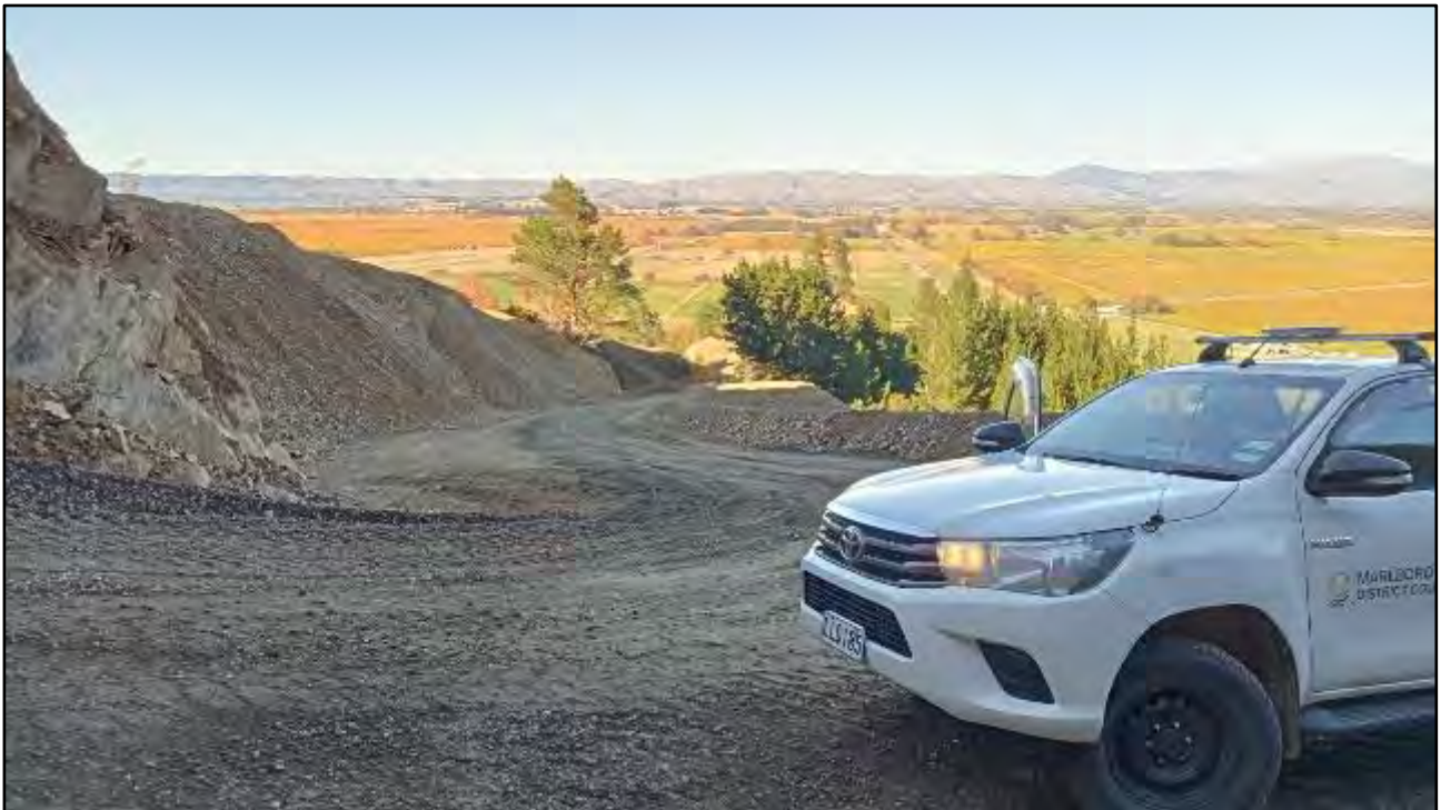
Figure 12 –Pukaka Quarry haul road completed.
