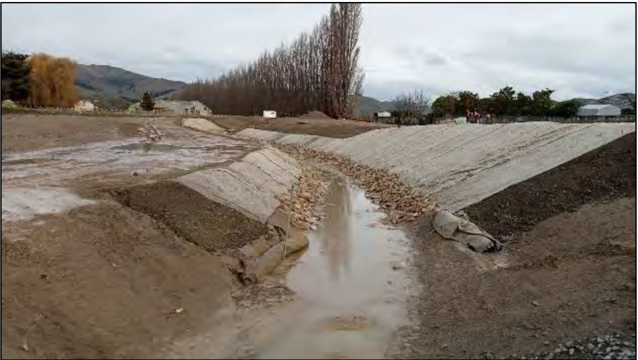
Figure 3 –Town Branch Drain realignment earthworks complete and landscaping underway.
