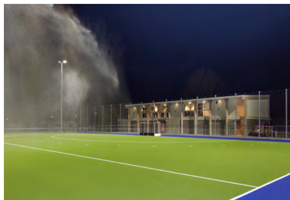
Fig 2 – Completed Hockey Turf
