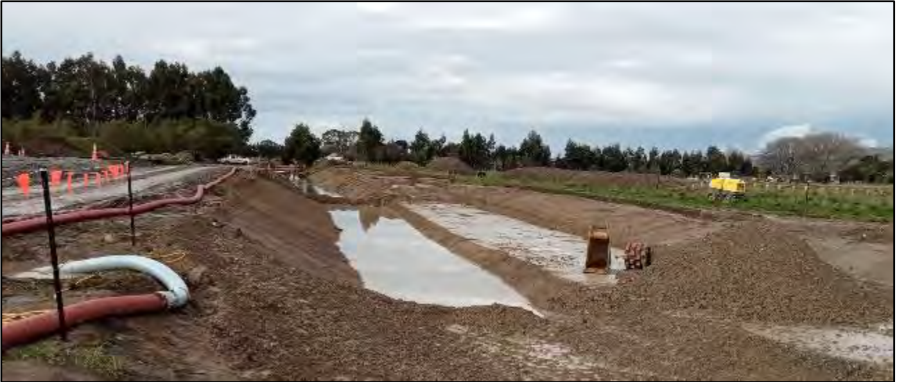
Figure 4 –Town Branch Drain widening underway.
