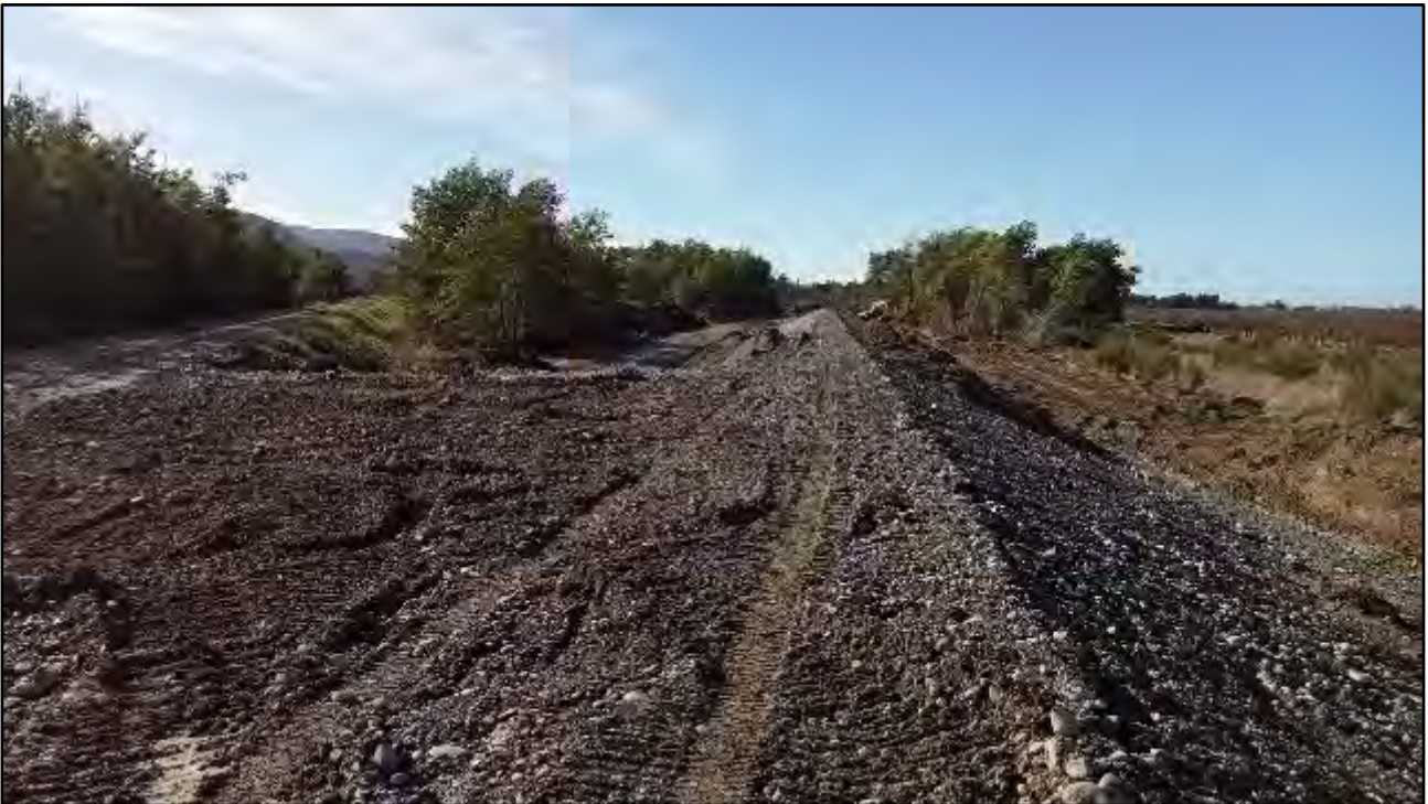
Figure 5 – Conders stopbank gravel core of new stopbank completed in late May.
