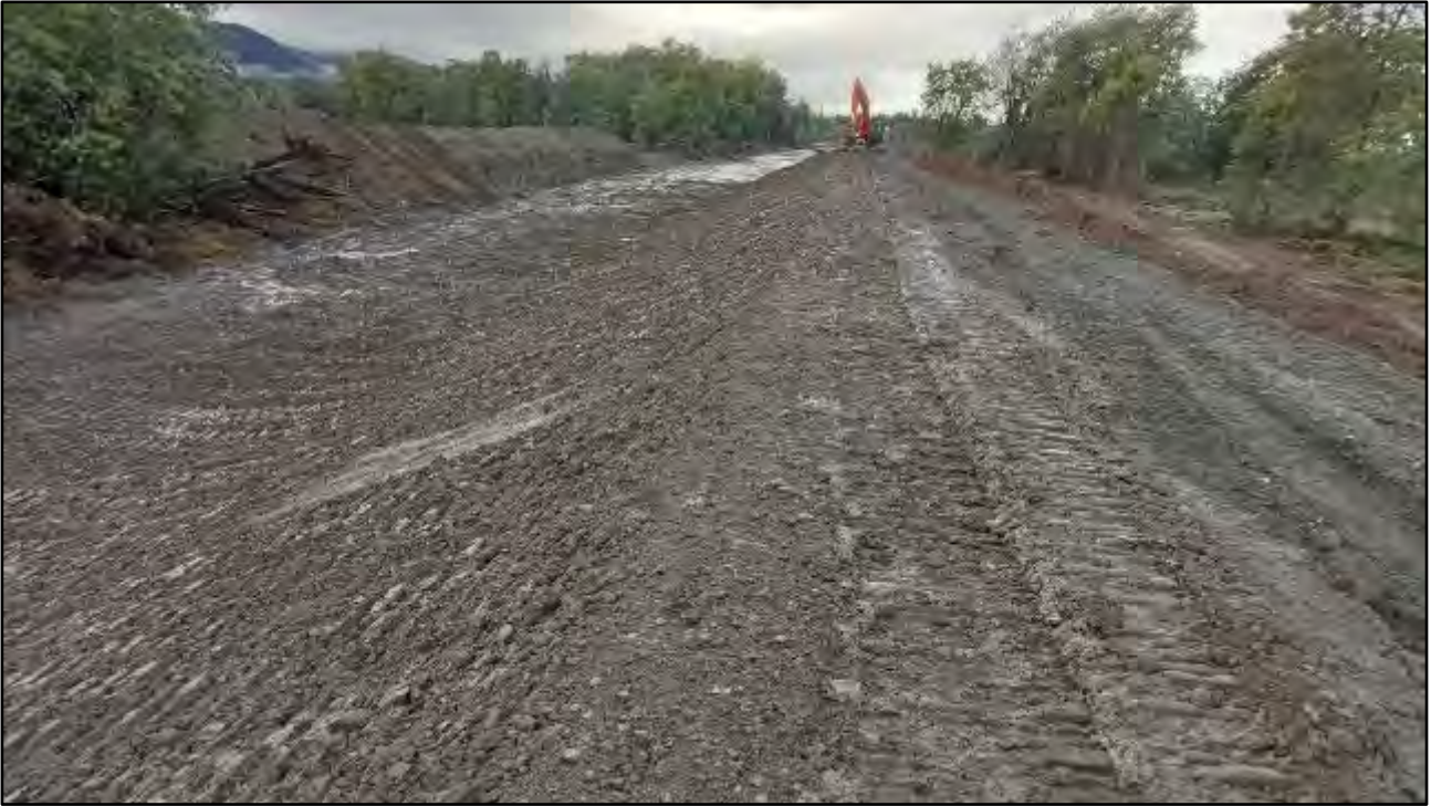
Figure 6 – Conders stopbank filter and facing layers completed mid-June in wet conditions.
