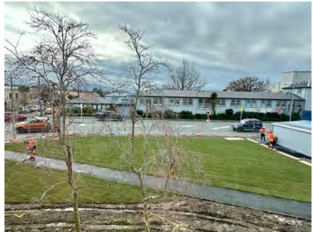
Fig 9 – Former MAG site development, asphaltting
