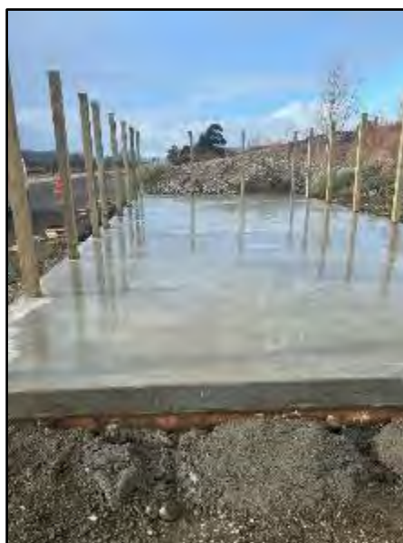
Figure 3 Awatere Valley Remote Transfer Station during construction
