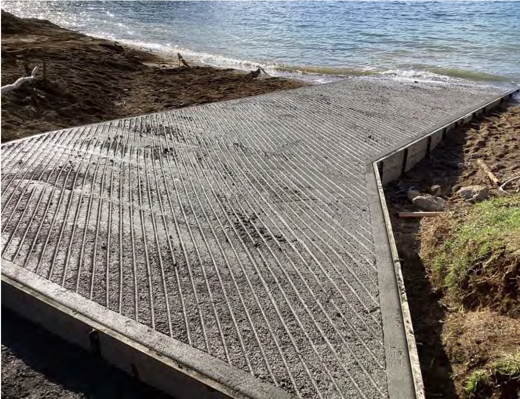
New boat ramp surface at French Pass – 30 June 2024.
