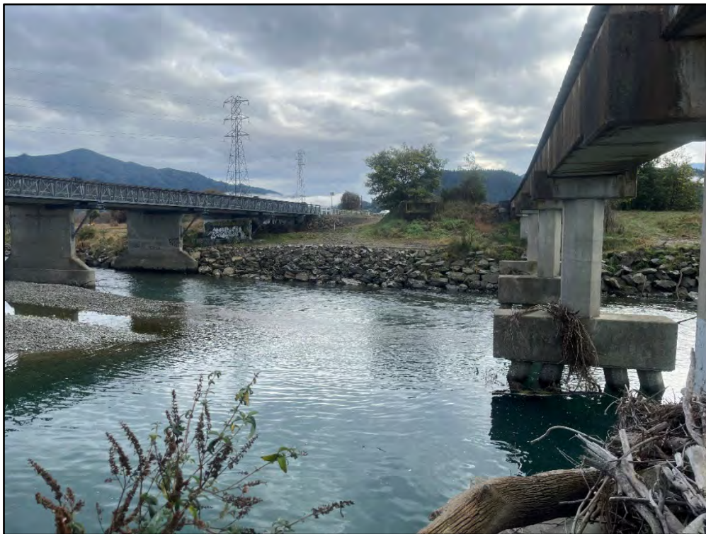
7 - Wairau Diversion Rockwall repairs
