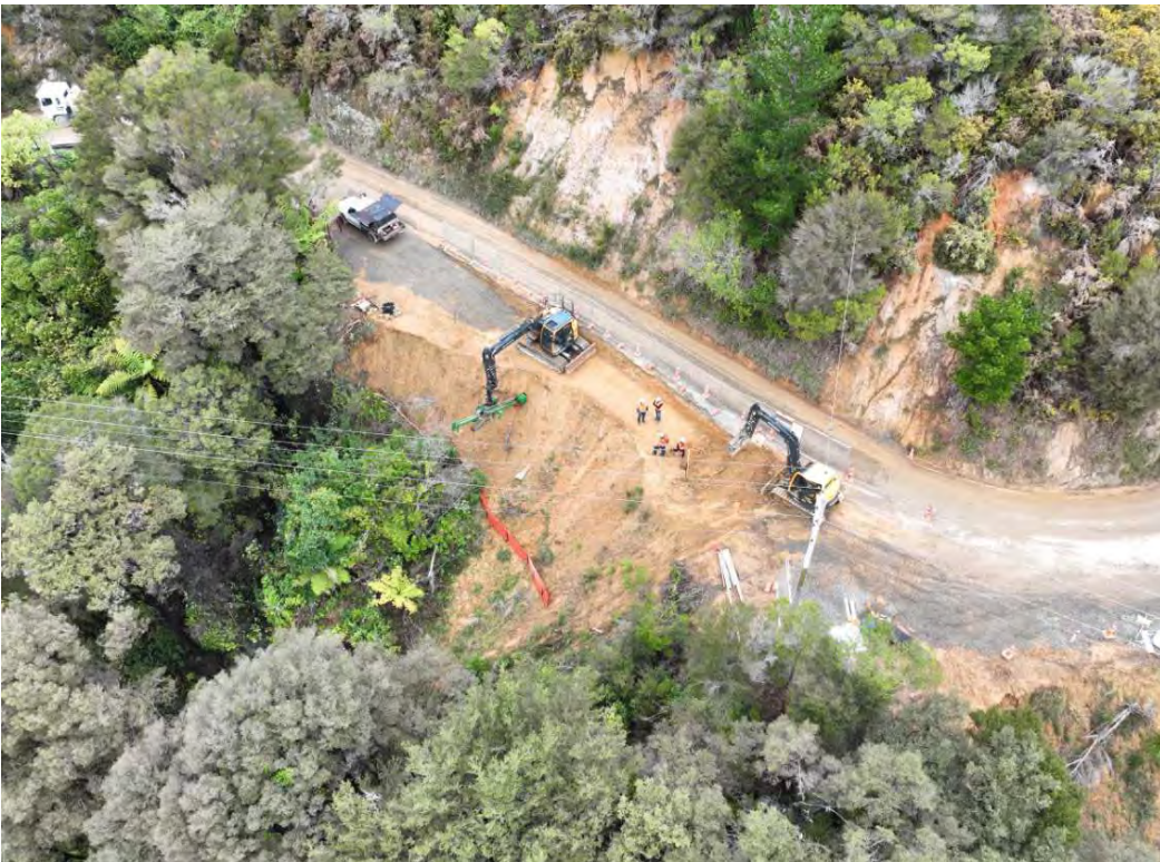
Anchor drilling for the new wall on Queen Charlotte Drive (716-03677) – 25 June 2024
