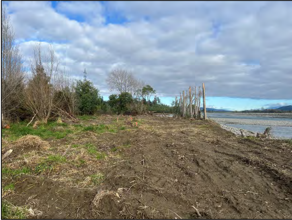
6 - Above SH6 TRB Bank repair works
