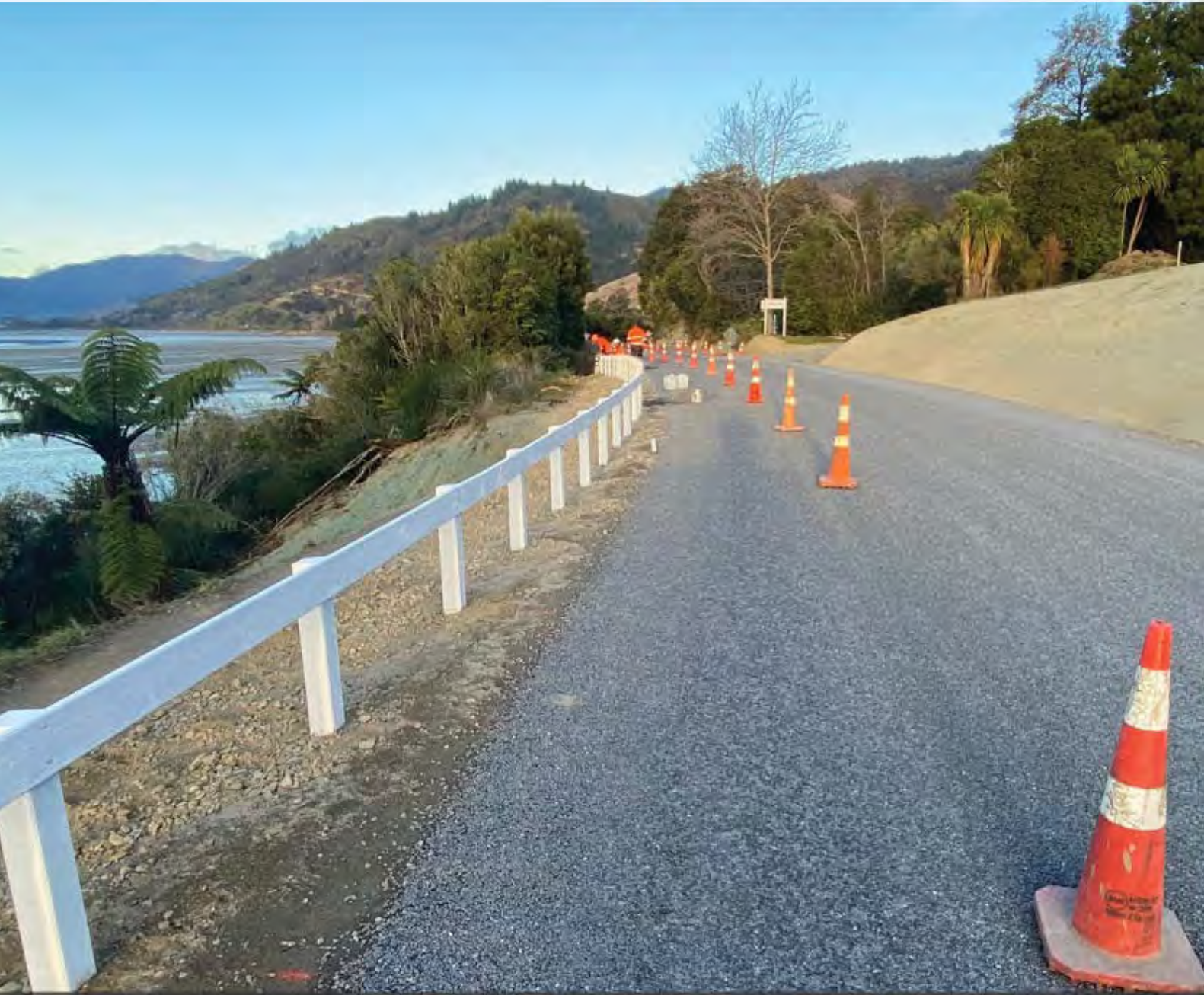
Sounds Road - Progress photo
