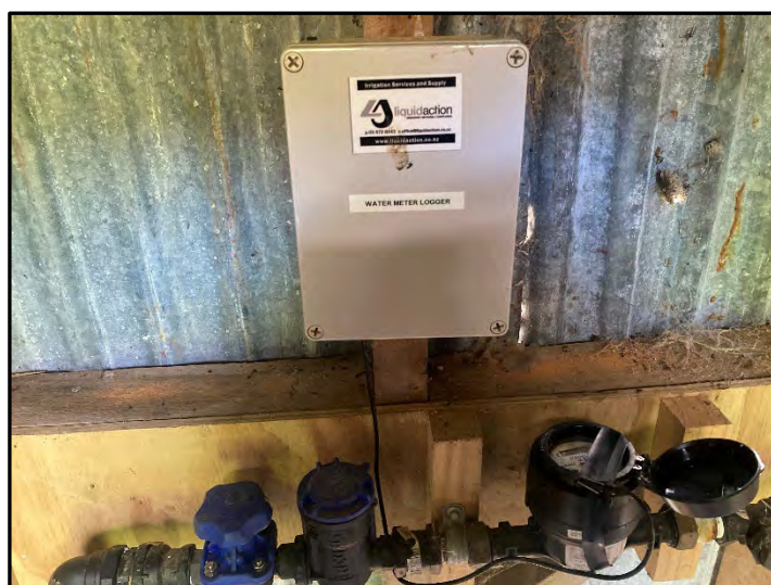
Water meters and logger at Carluke Domain
