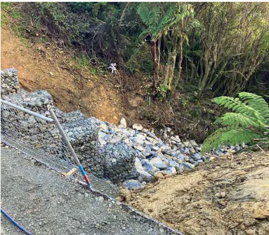
Gabion spill way wall and rock armouring at Cullens Point – 12 June 2024
