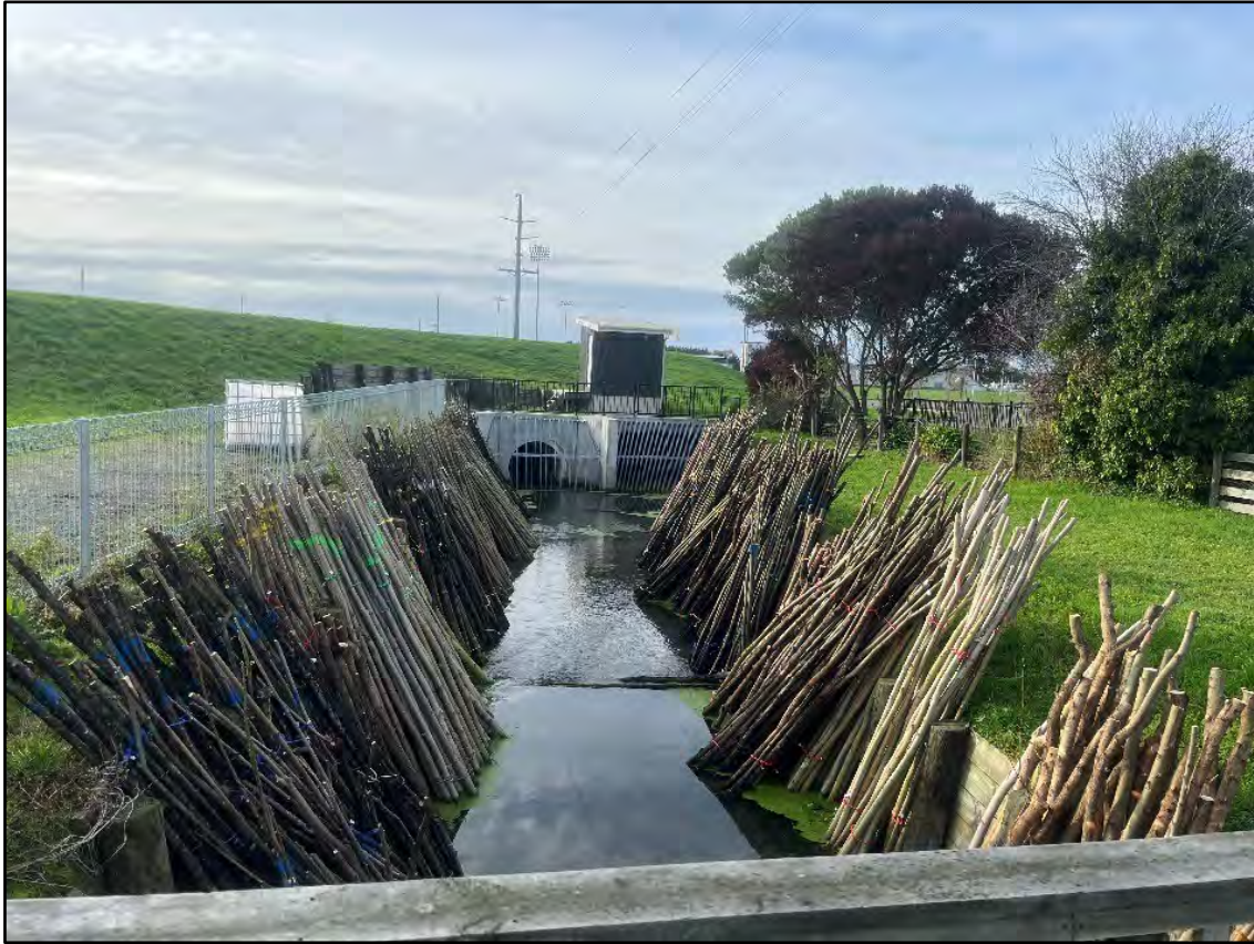
9 - about 2500 poles harvested and stored in creek
