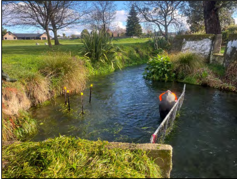
12 - Debris collector at Murphys Creek confluence
