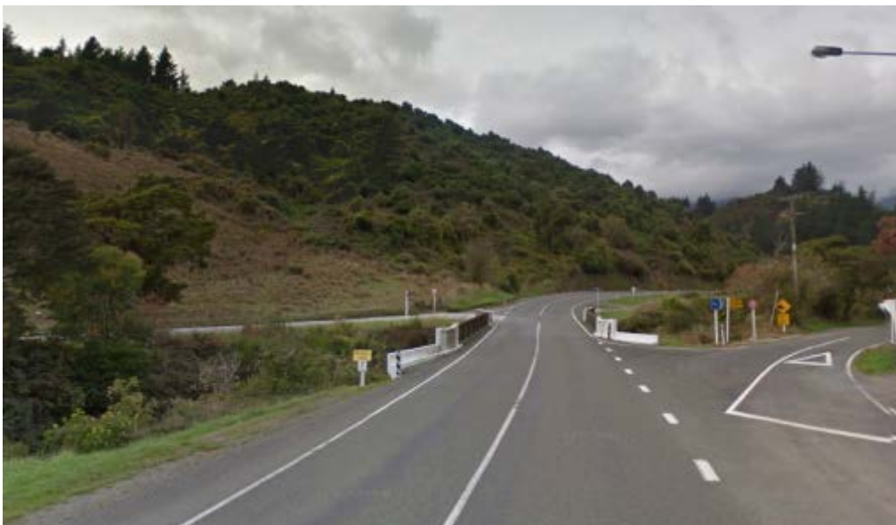
SH6 Teal River Bridge at the base of the Whangamoia travelling towards Blenheim
