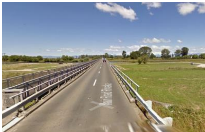
SH60 Motueka Bridge approaching from Riwaka
