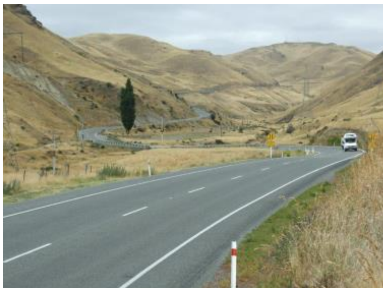
Puka Puka Weld Pass SH1, Marlborough
