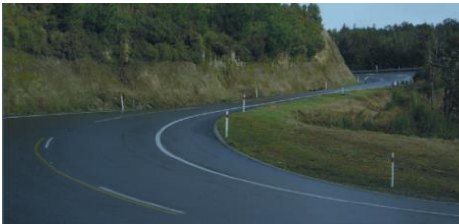
SH6 Hope Saddle approaching from the North
