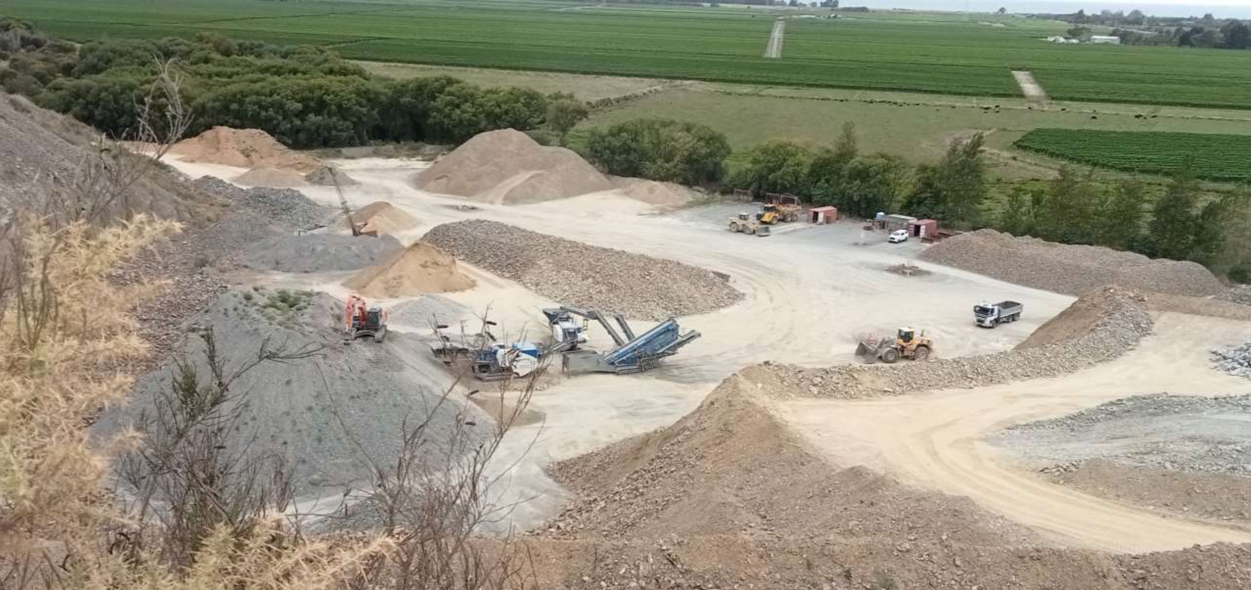
2024 Pukaka Quarry Development
