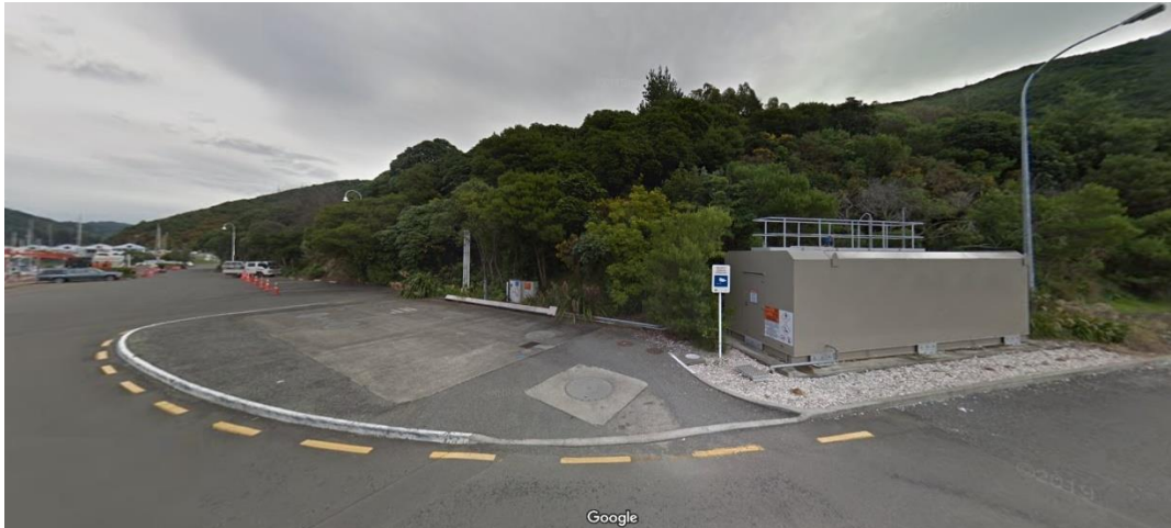
Figure 8: Existing hardstand and fuel tank at Jetty 6W
