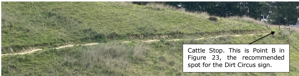
Figure 22. The section of Easy As immediately beyond the first cattle stop has a strange and unnecessary wavy surface configuration.
