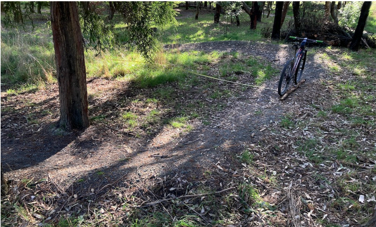
Figure 45. This is typical of the turns on Wiggles; large-radius but not necessarily grade-compliant. They are – appropriately – minimally bermed and while they might be challenging for their usual target riders (Beginners), they will be easy for racers in the secondary school champs. In places however, riders will need impact protection if they overshoot these corners at race speeds.
