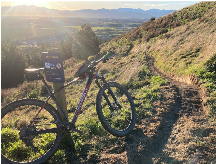
Figure 25. The entry, and the first few metres of Mogwai. Recent hand-completed work has smoothed the track but it's only 300-500mm wide. The standards vary but with this side slope, it needs to be 400-600mm.
