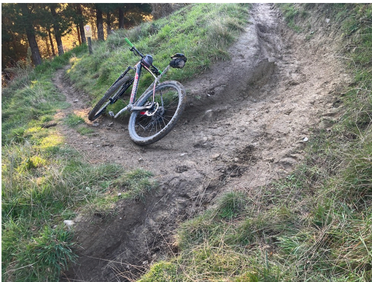
Figure 26. The badly eroded, tight and steep lower (second) corner on Mogwai. Some work could restore this to Grade 5 but probably not Grade 4, without realignment. Most importantly, the trail is eroding badly and is not sustainable.
