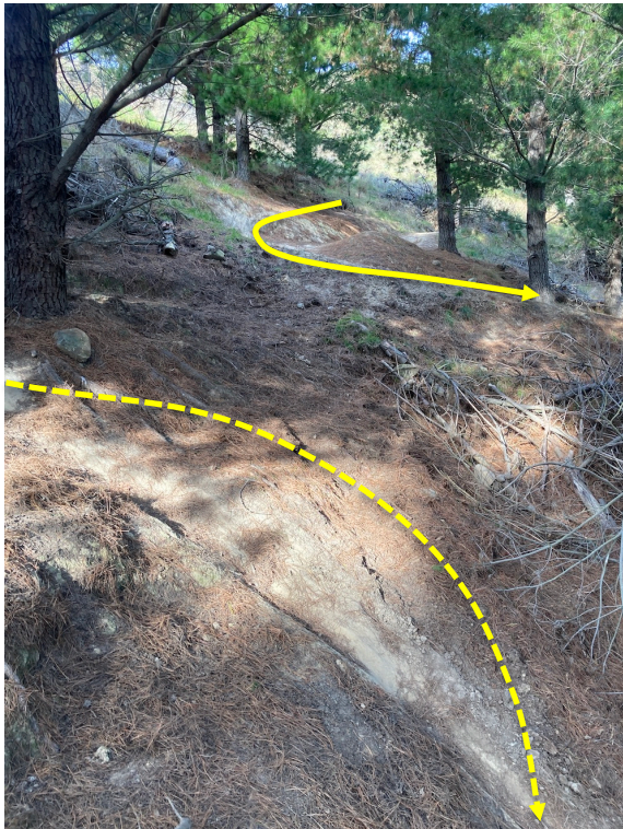
Figure 42. Detail of the second (RH) corner on Lamb Chops (dashed line). It is essentially unformed and very rooty, and crosses the fall line at 15-20° - Grade 5. Lamb Chops is not suitable for the upcoming event but if it is used, we'd recommend entering the trail from Captain Slapstick (above, yellow arrow) to avoid the first two unformed corners.
