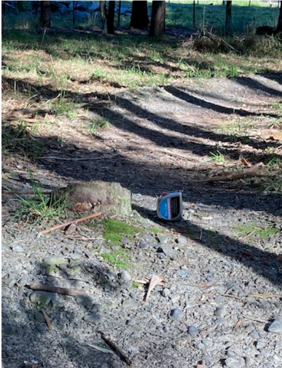
Figure 44. Protruding timber on Wiggles Trail (with tape measure for scale).
