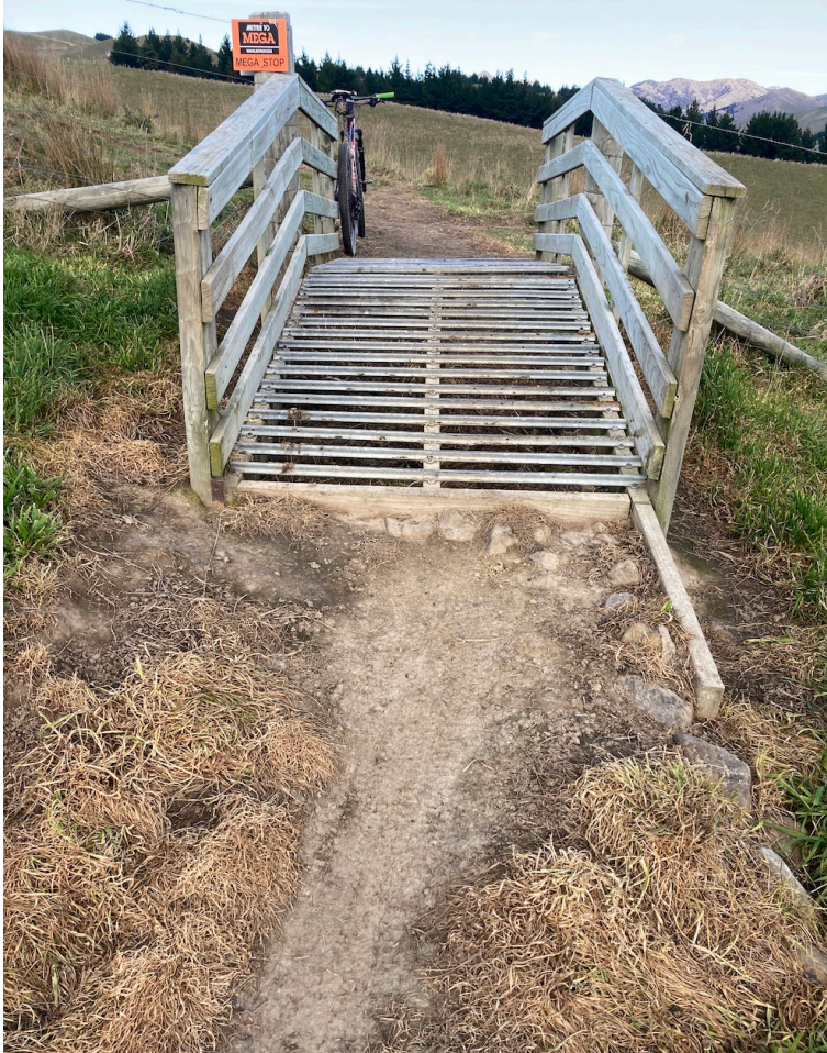
Figure 13. One of the trickier cattle stops heading uphill on Scenic Route (Northern)
