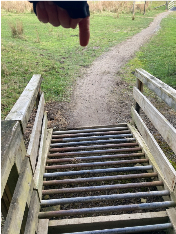
Figure 14. The (downhill) approach to one of the cattle stops on Stockyard. The corner is not quite finished when riders have to cross an obstacle with constricting, vertical sides that is narrower than the nominal minimum required for the track: 1.5m.
