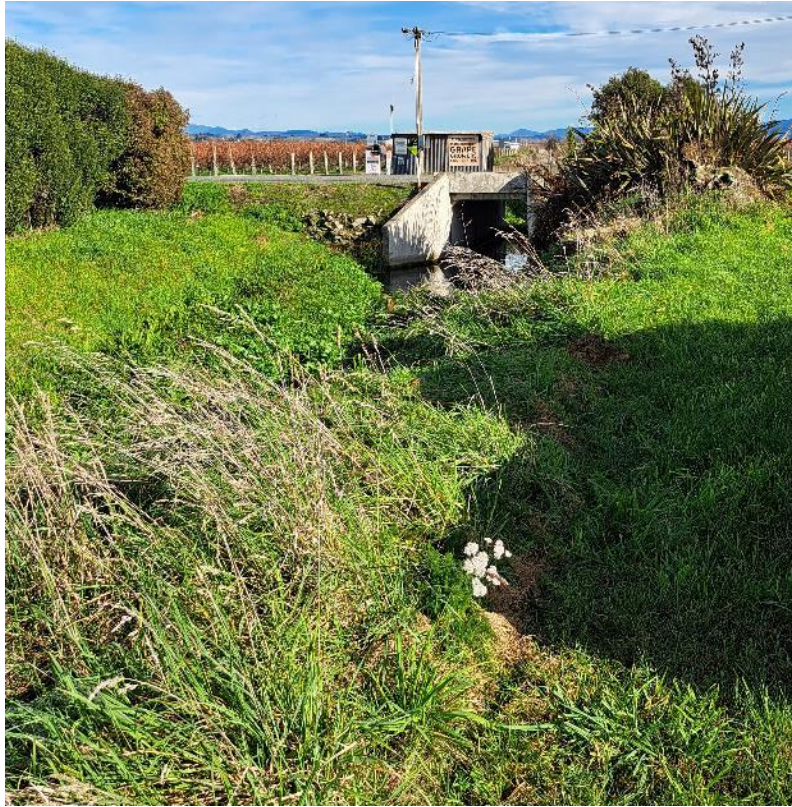
Figure 3-10 Fairhall Co-op Drain at Bells Road (facing up-channel, 27/06/2023)
