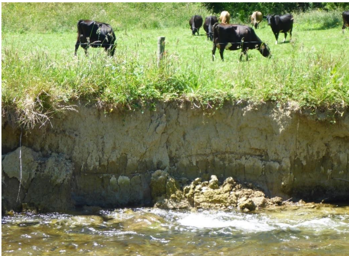
Figure 2-3: Example of streambank erosion in the Rai River catchment (December 2016). Photo: A. Swales, NIWA.
