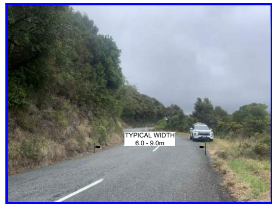
TYPICAL ROAD EXAMPLE: DESIGN VEHICLE 1: AUCKLAND TRANSPORT - TRUCK - 12.6m - NO HITCH DESIGN VEHICLE 2: AUCKLAND TRANSPORT - 85m - CAR WITH CARAVAN CHECK VEHICLE: RTS-18 SEMI TRAILER (17.9m)
