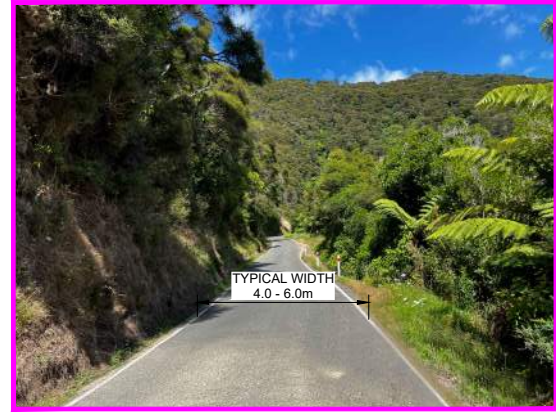
TYPICAL ROAD EXAMPLE: DESIGN VEHICLE: NONE CHECK VEHICLE: 17.9m SEMI TRAILER (RTS-18)
