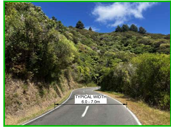
TYPICAL ROAD EXAMPLE: DESIGN VEHICLE: AS/NZS 2890.1:2004 B99 VEHICLE CHECK VEHICLE: 17.9m SEMI TRAILER (RTS-18)
