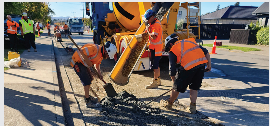
Contractors working in McLauchlan Street
